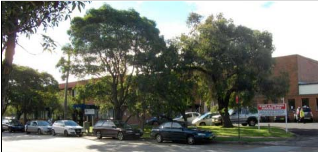
Figure 2: The existing building on the site
